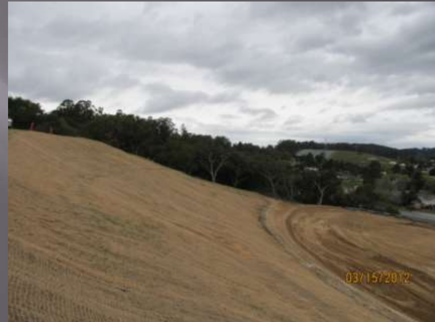
2 Ft Slope Benches (Every 15-30 vertical Feet)
