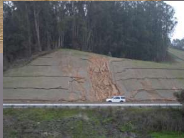
Top of Cut Ditches
